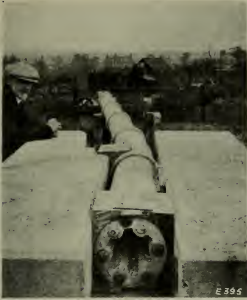
"MARRIOTT" REINFORCED CONCRETE TELEGRAPH POST.
